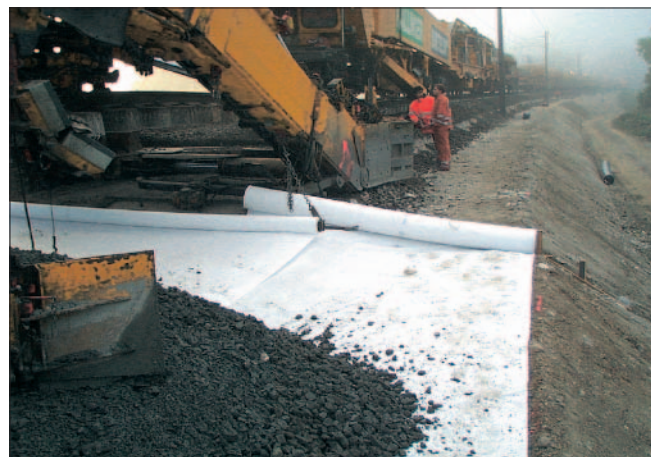
Figure 10: The standard drawing specifies that the geotextile must cover the lower edge of the track-bed layer
