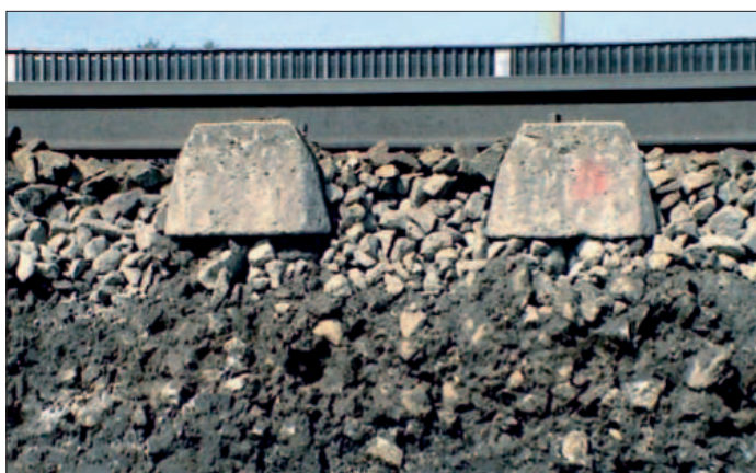
Figure 5: Track ballast after 27 years of operation with approx. 500 million load tons
