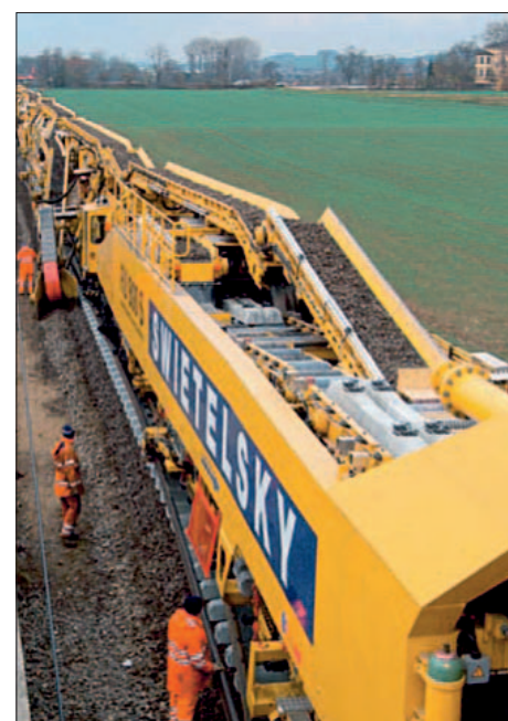
Figure 8: RU 800 S – picking up ballast from the shoulder
