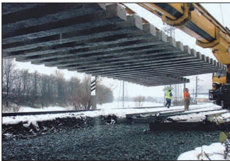
Fig. 8: Dangers caused by suspended loads
