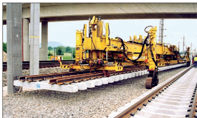
Fig. 4: The “PK1” gantry-crane point-laying system
