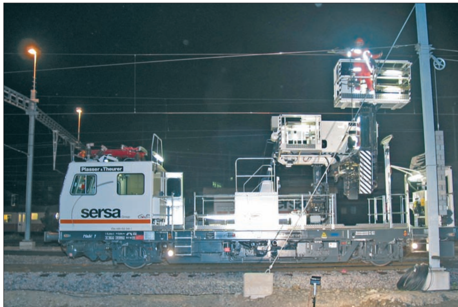
Fig. 11: FGW 10.010 catenary during assembly work in Zurich main station
