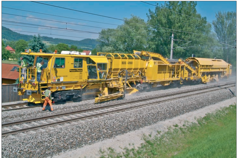
Fig. 8: Better distribution of ballast using the BDS system
