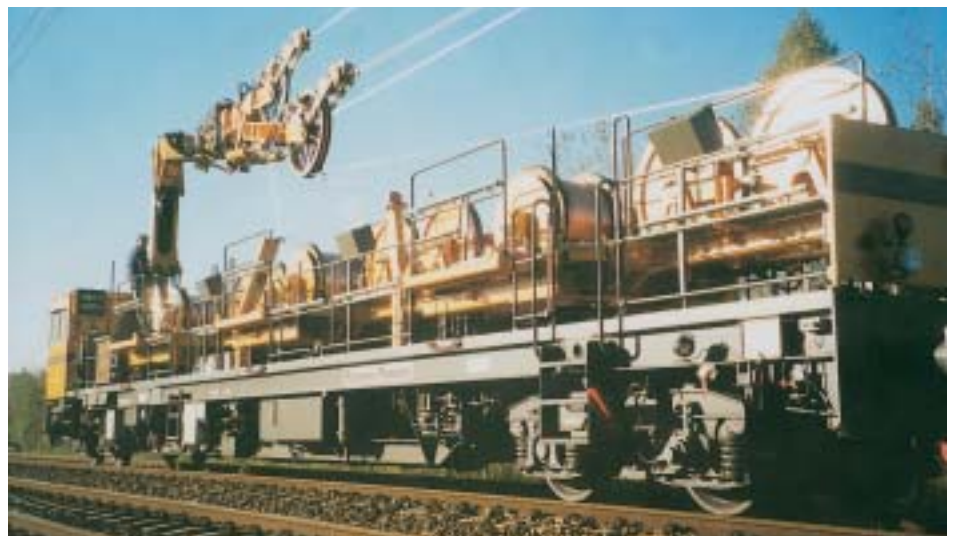
Fig. 3: Catenary-installation machine for handling three cables simultaneously
