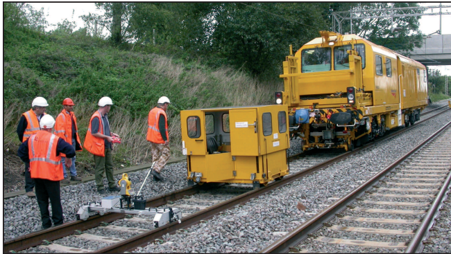
Fig. 3: EM-SAT track survey car on Network Rail, United Kingdom
