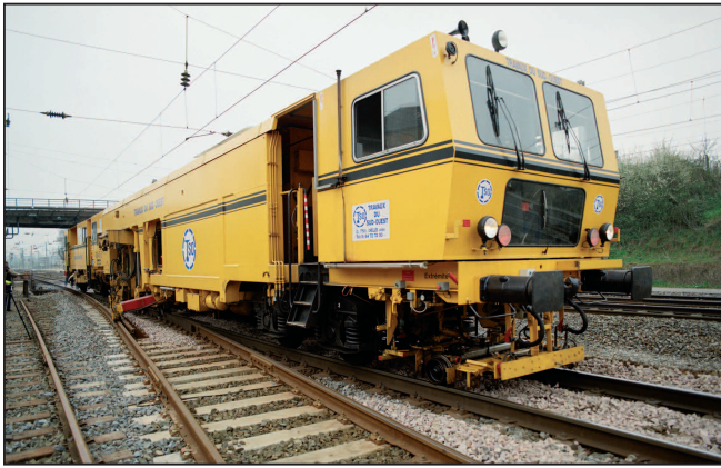
Fig. 8: Tamping of a high-speed switch in France
