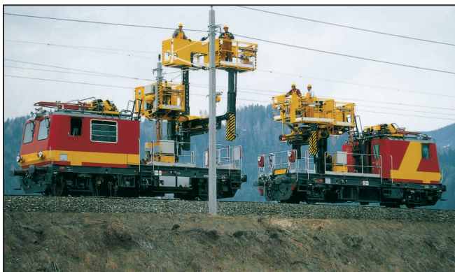
Fig. 3: Assembly tower cars (MGW) with three independently-controlled column elevating work platforms
