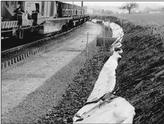
Fig. 12: Example of a finished protective layer with drainage (line Linz - Salzburg)
