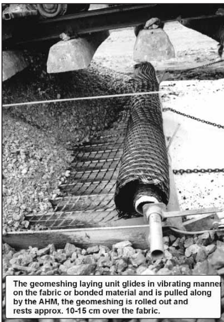
Fig. 3: Installation of geomeshing
