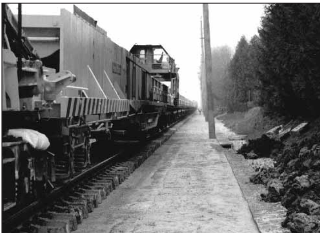
Fig. 4: Example of a finished protective layer (line Wels - Passau)
