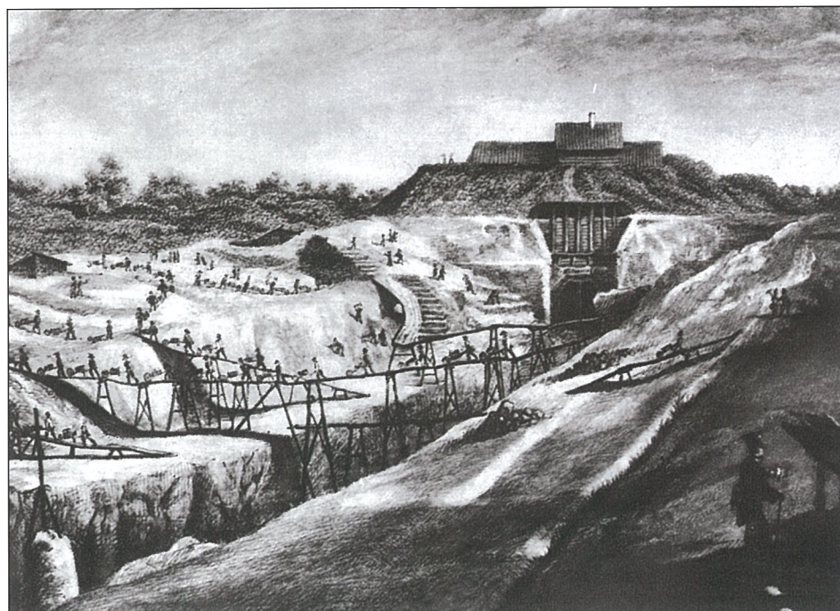
Fig. 5: Earth transport on wooden tracks during the construction of the first railway tunnel near Oberau which was built by Freiberg miners between 1837-1839.
