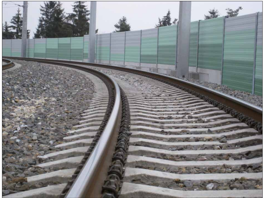
Fig. 11: Curve with HD sleepers at Sankt Pölten
